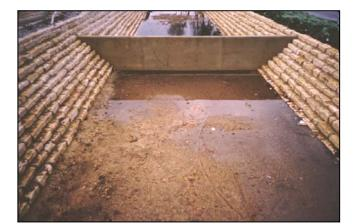
**Description**: Surface sand filters are multi-chamber structures located above ground that are designed to treat stormwater runoff through filtration, using a sediment forebay, a sand bed as its primary filter media and, typically, an underdrain collection system.
